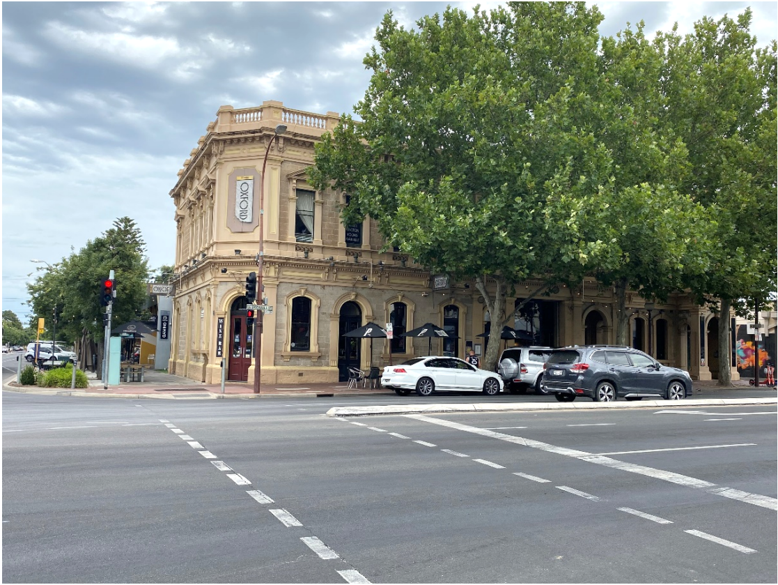
Figure 3.6 – Oxford Hotel, looking west from corner of Tynte and O'Connell Streets
